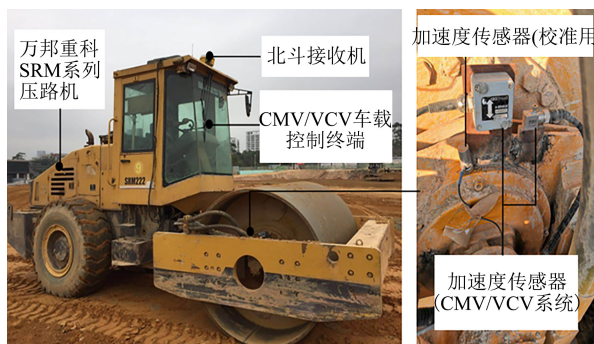
图1 现场试验碾压设备 Fig.1 Field test rolling equipment
