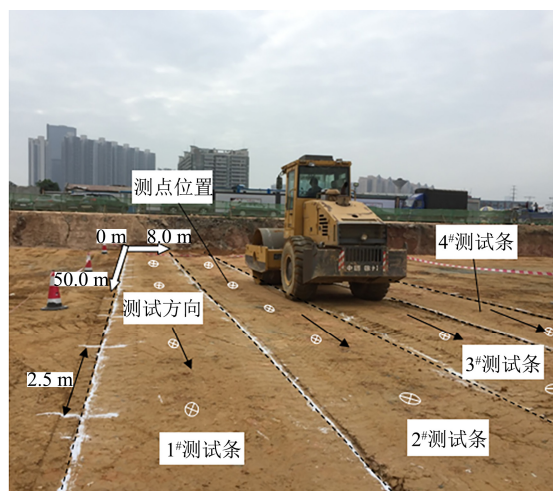
图2 测试条布置 Fig.2 Layout of test strips
